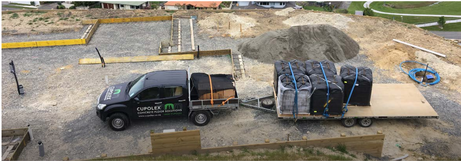
GOOD SITE PREPARATION
