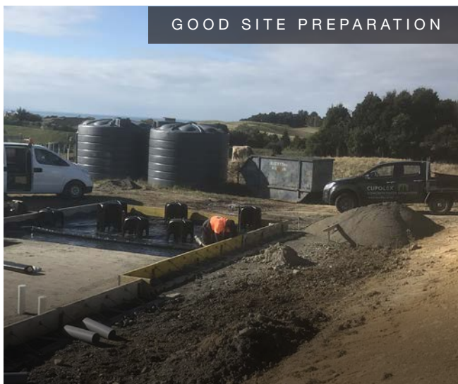
COMPACTED AND READY TO GO
