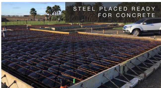
THICKENING BEAM WITH RE-ENTRY CORNERS
